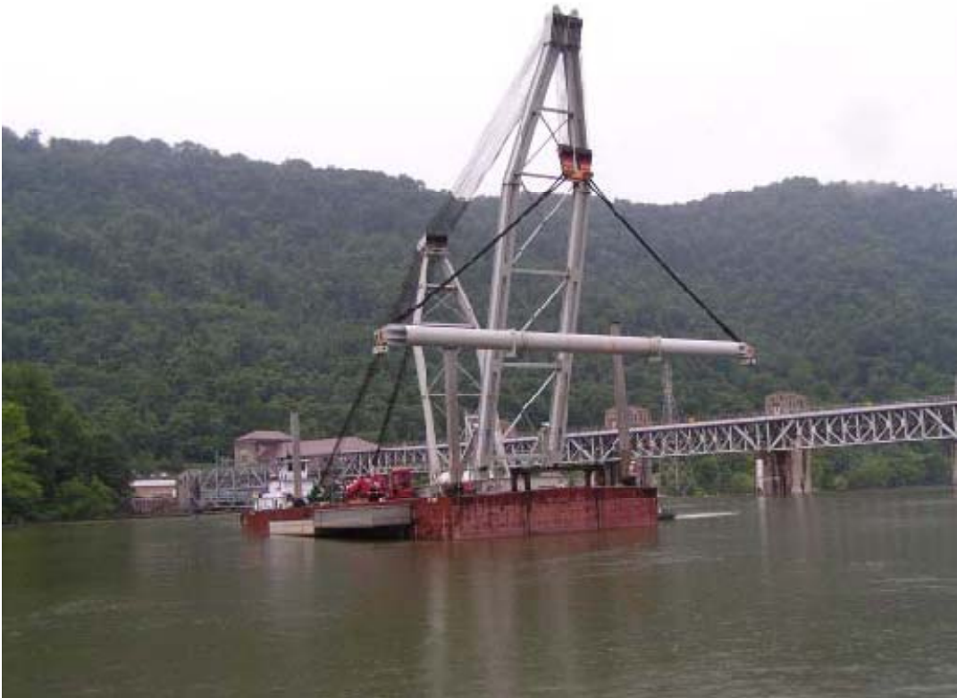
Figure 1.5 Lifting the Post-tensioned Beams at London Lock (courtesy of Huntington District)
