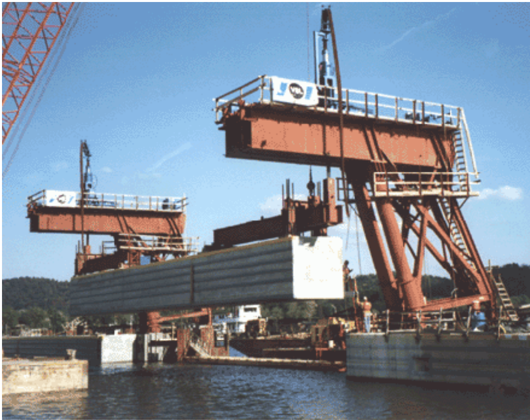
Figure 1.7 Winfield Lock Approach Wall Beam at Placement (courtesy of Huntington District)
