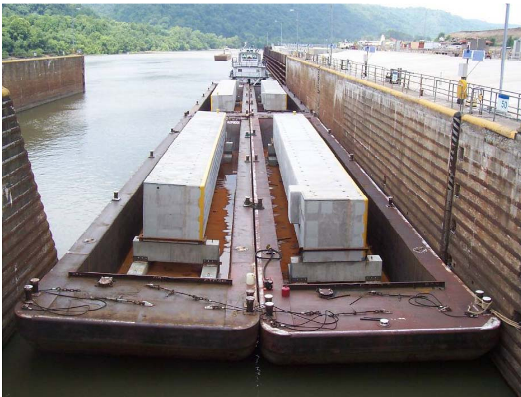
Figure 1.3 Transporting the Post-tensioned Beams to Marmet Lock (courtesy of Huntington District)
