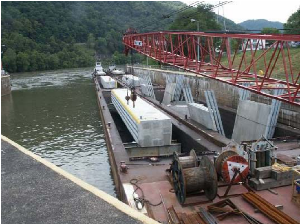
Figure 1.6 Transporting the Post-tensioned Beams to London Lock (courtesy of Huntington District)
