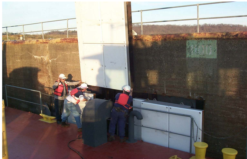
Figure 6.4. Insertion of middle prototype panel into wall fendering system
