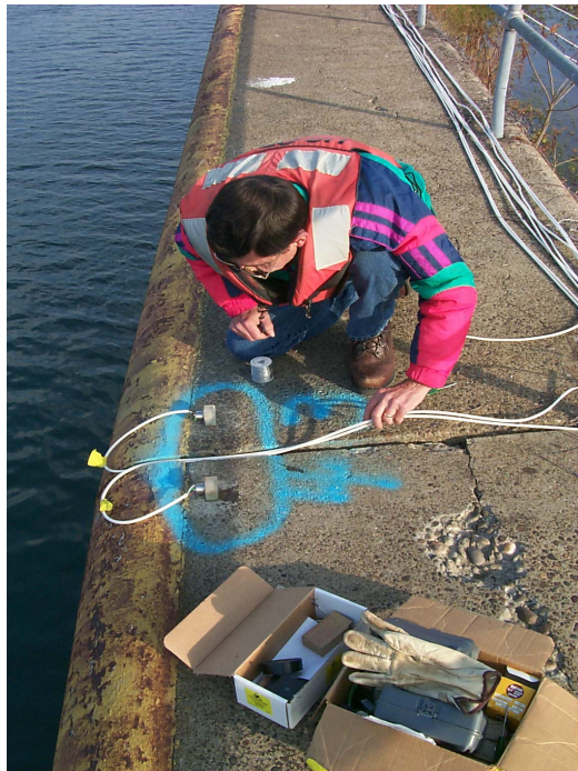
Figure 5.22. Installation of accelerometers on lock wall
