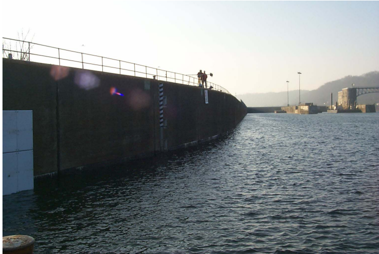
Figure 3.2. Upper guide wall at Gallipolis Lock (Note: As reference, prototype fenders are on the left; lock chambers are straight in the distance; and the dam is on the right)
