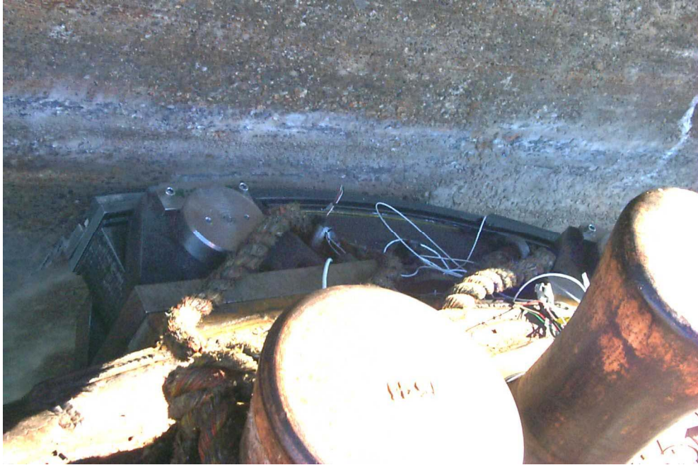
Figure 5.12. Load beam impacting guide wall
