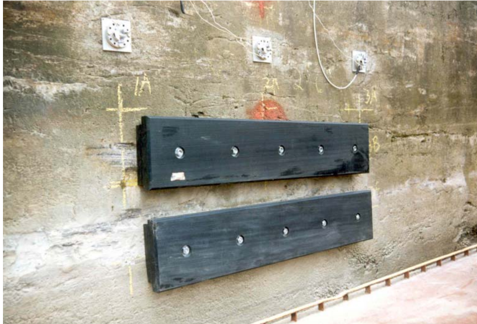
Figure 20. Final setup of UHMW bumpers
