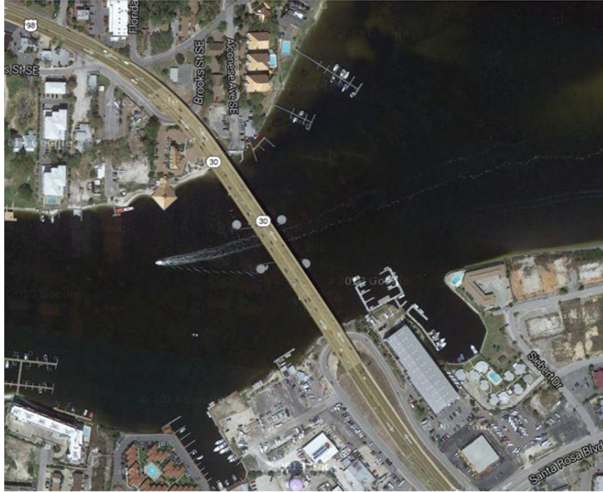
Figure 5.5 Curvature of waterway near Brooks Bridge (Source: Google)
