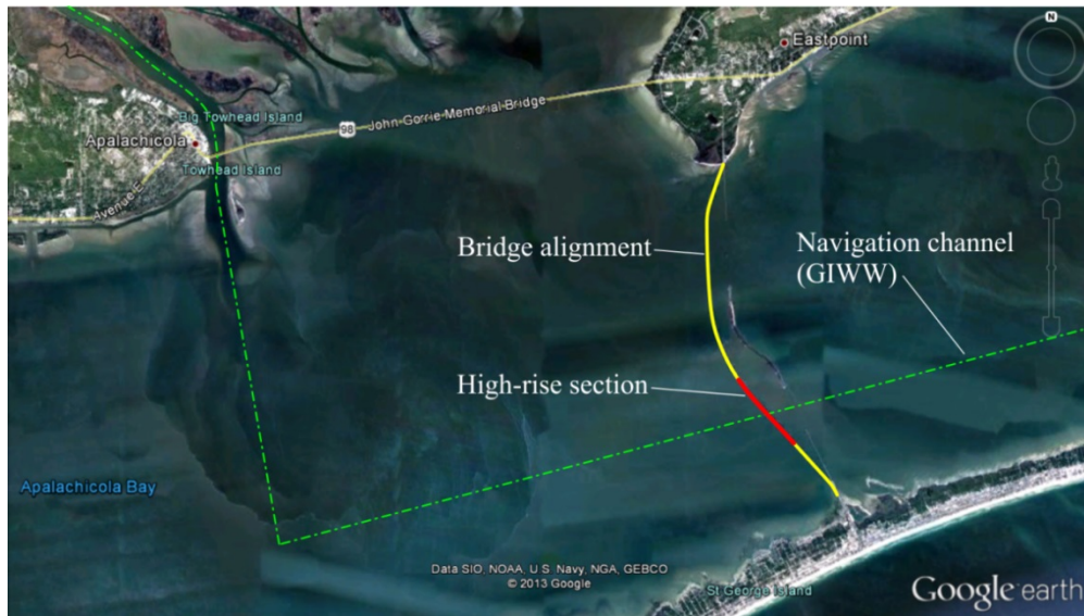
Figure 5.10 Bryant Grady Patton Bridge (SR-300) spanning Apalachicola Bay, Florida (Consolazio et al. 2014)
