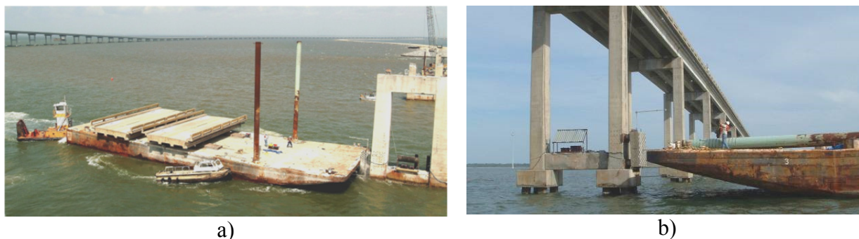
Figure B.2 Full-scale barge impact experiments at St. George Island, Florida: a) Stand-alone pier impact (superstructure removed), and b) Intact bridge impact (Source: Consolazio et al. 2005)
