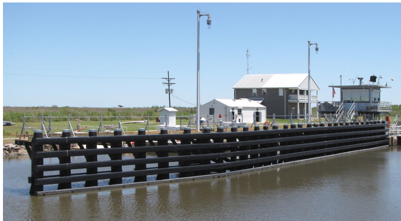
Figure 1.4. Flexible timber guide wall structure (Photo credit: U.S. Army Corps of Engineers)
