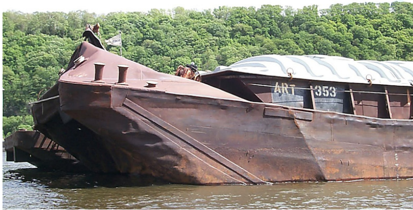
Figure 2.7. Severe bow deformations from barge impact at Mississippi River Lock and Dam No. 9. (Photo credit: U.S. Army Corps of Engineers)
