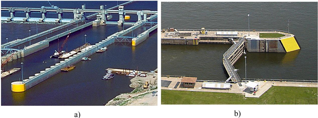
Figure 3.1. Primary types of bullnose structures considered: a) Circular geometry; b) Mississippi sloped-V geometry (2:1 vertical-to-horizontal slope)
