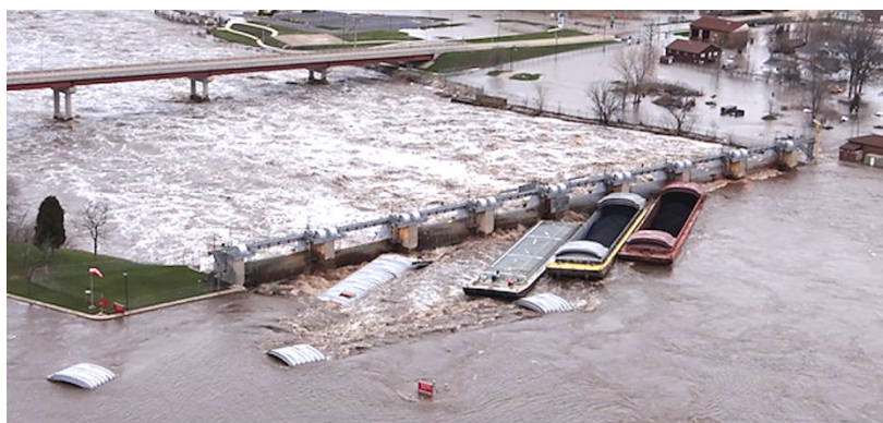
Figure 1.3. Individual barges jammed against Marseilles, Illinois Dam after breaking free from remainder of barge flotilla (2013) (Photo credit: U.S. Coast Guard)
