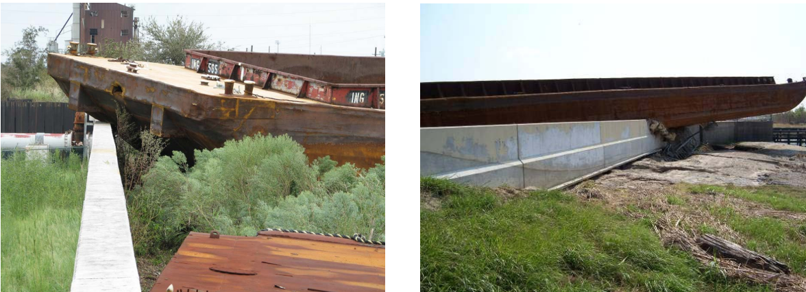
Figure 1.1 Aberrant barges that impacted New Orleans area floodwalls during Hurricane Katrina (Source: U.S. Army Corps of Engineers).
