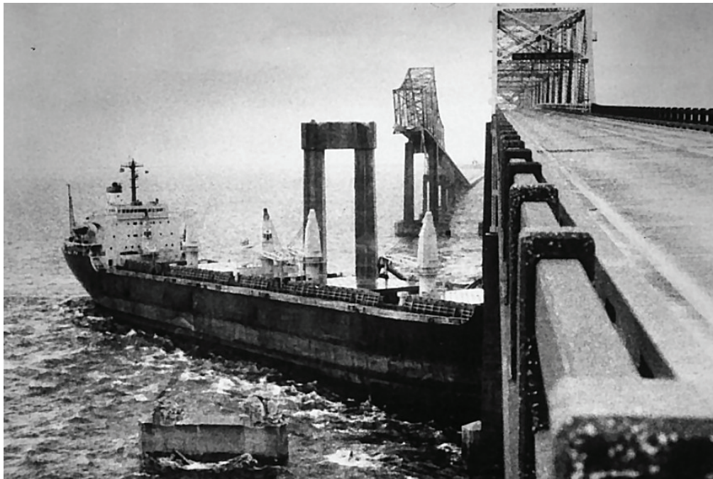
Figure 2.1 Collapse of the Sunshine Skyway Bridge in Tampa, FL (1980) due to ship collision
