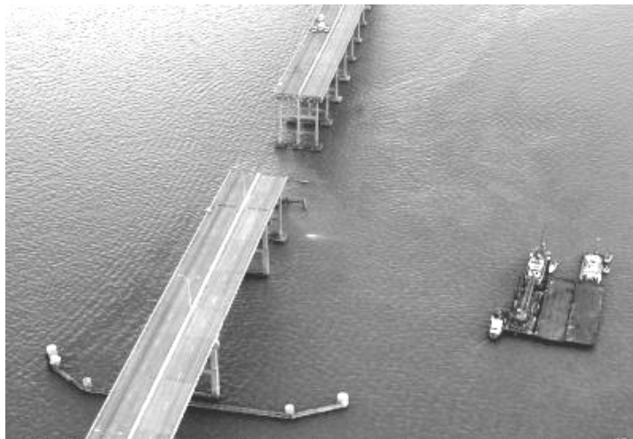
Figure 2.3 Collapse of the Queen Isabella Causeway Bridge in Texas (2001) after being struck by a barge flotilla
