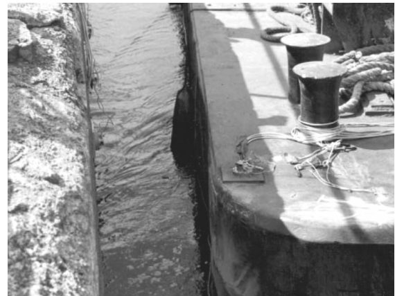
b) Sensors at impact corner of barge
