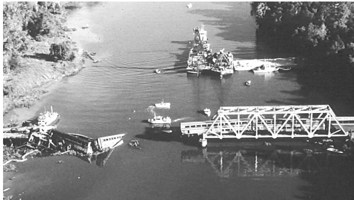
Figure 2.2 Failure of the Big Bayou Canot railroad bridge in Alabama (1993) after being struck by a barge flotilla
