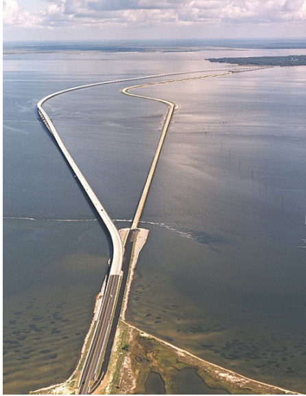
Figure 3.4 Aerial view, looking north, of St. George Island Causeway Bridges (Barge impact tests were conducted on the old bridge, at right)
