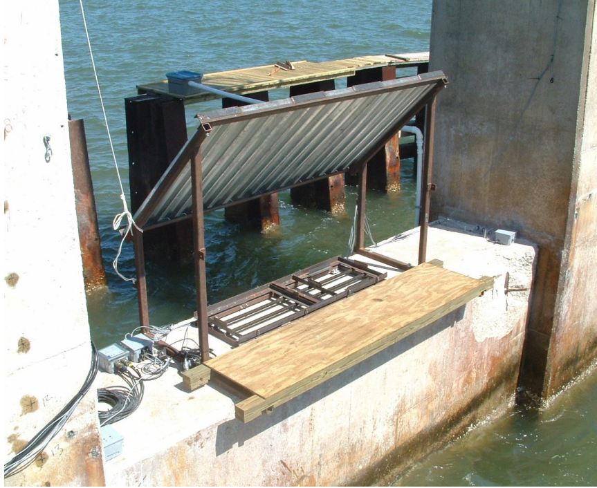
Figure 6.17 Shock isolation sled and debris shelter for DAQ and DC cases installed on Pier-1
