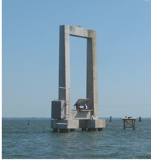
Figure 5.9 Pier-3 isolated for series P3 tests
