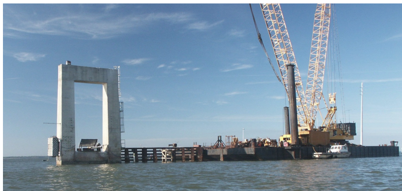
Figure 5.3 Stationary barge with winches spudded down on east side of Pier-1
