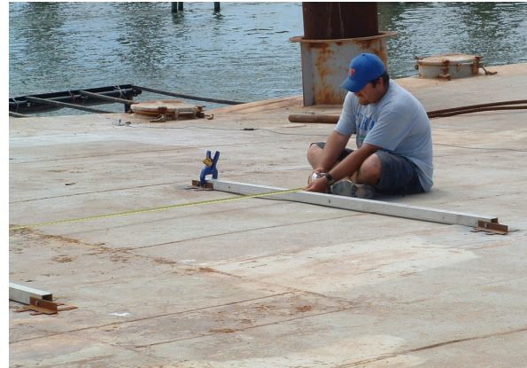
b) Recording distance measurements at datum beam
