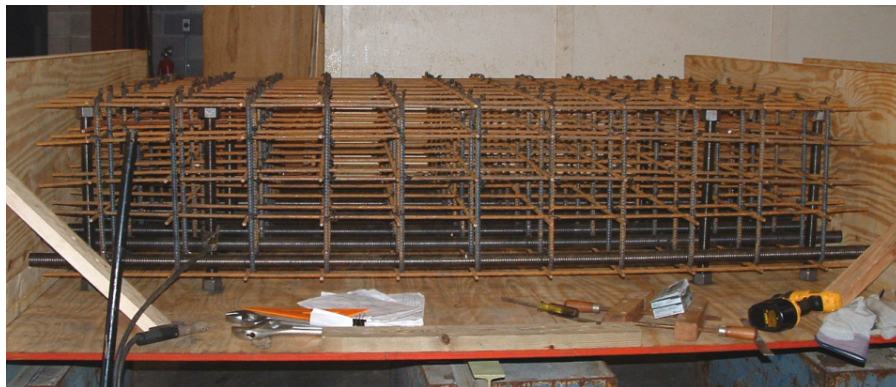
Figure 6.23 Internal steel reinforcing used in impact blocks
