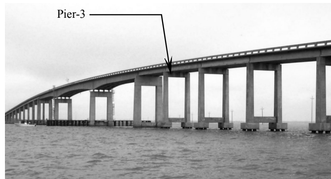
Figure 10-11 Pier-3 in relation to entire bridge structure (view looking North)
