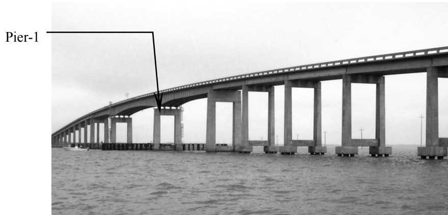
Figure 10-3 Pier-1 in relation to entire bridge structure (view looking north)
